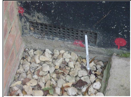
Air brick acting as a gutter
