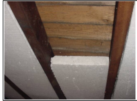
Close boarding with insulation beneath it
