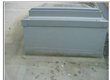
Pre-forming around the roof window
