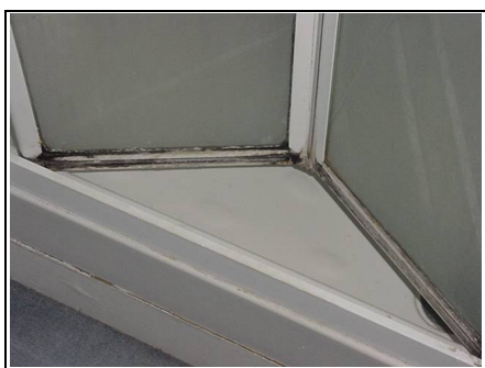
Mould to bathroom
