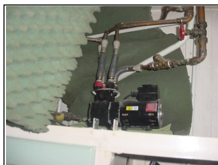
Pump hidden behind insulation in study
