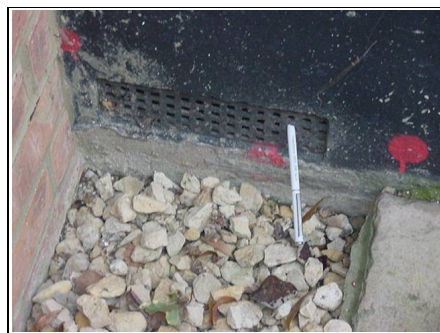
Airbrick acting as a gutter
