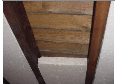
Part of the insulation removed to see the close boarding
