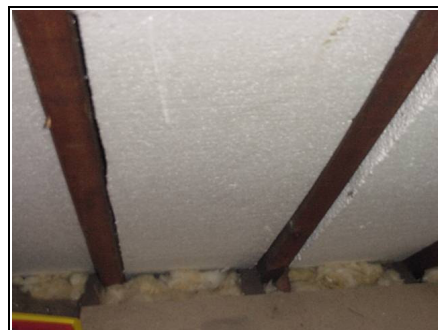
Insulation board in roof space
