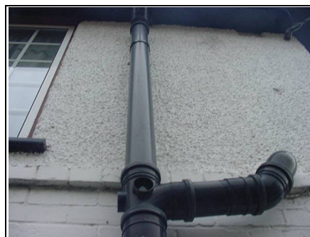
Bend in soil and vent pipe
