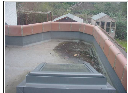
Ponding to flat roof
