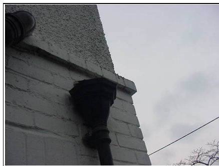
Cast iron gutters and downpipe
