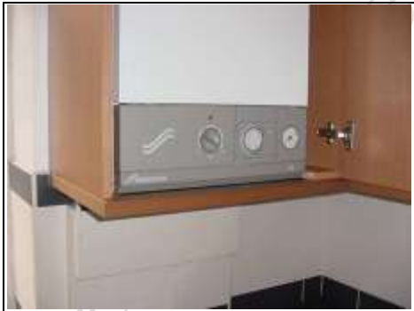
Wall mounted Worcester Boiler
