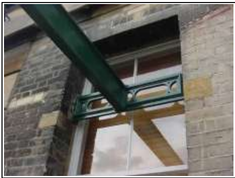
Unusual window with cast iron beam
