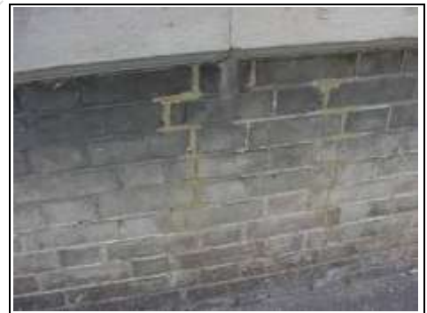
Repairs to cracking
