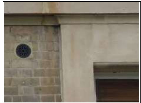
Vent for the gas boiler
