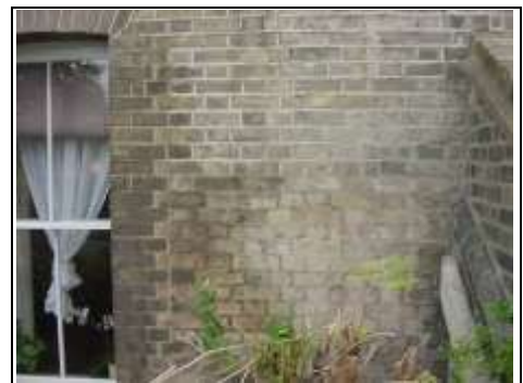
Wet area to flat below – right hand side of property
