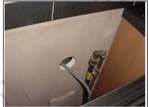
False wall / dry lining in the kitchen
