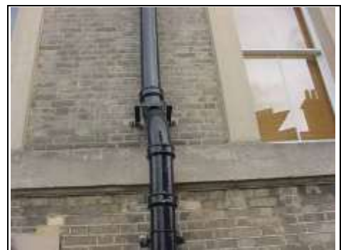
Possible asbestos downpipes
