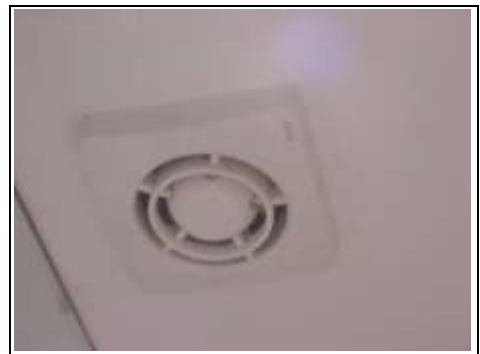
We recommend replacing this extract fan with a humidity controlled extract fan
