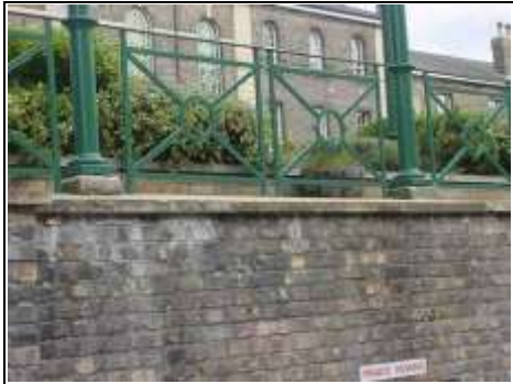
Retaining wall without weep holes
