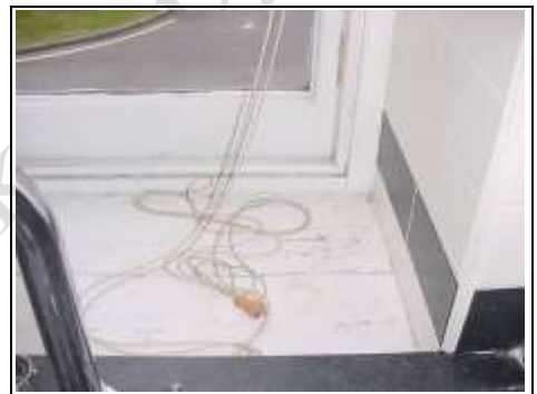
Kitchen window sill. Signs of condensation.
