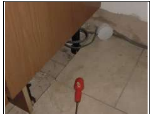
Tiled floor has been laid on the old floor and cut around the units
