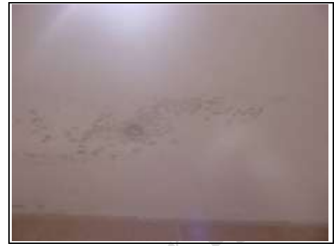
Mould in the bathroom
