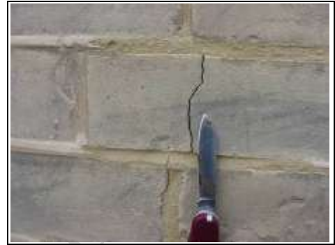
Vertical crack in the brickwork
