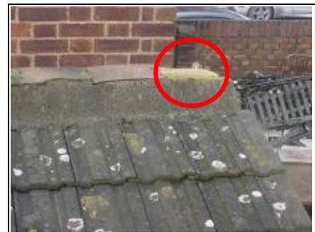
Missing tile on single pitch roof
