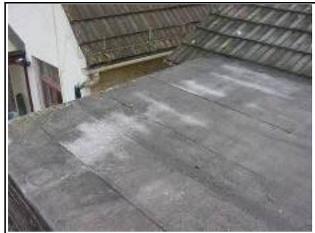
Rear flat roof with bitumen finish
