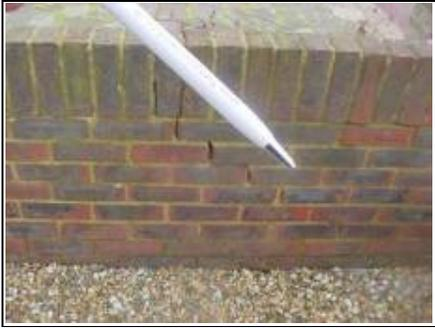
Step cracking in wall will need repairs.
