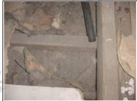
Lath and plaster ceiling visible from roof space
