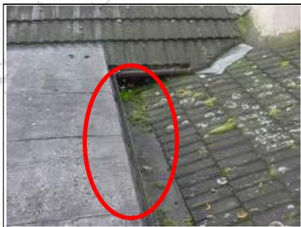
Hidden valley gutter where the flat roof meets the single pitch roof
