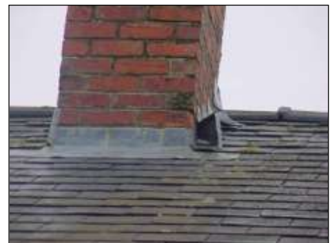
Chimney one showing lead coming loose, possibly some repointing needed
