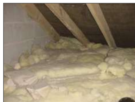
Roof insulation
