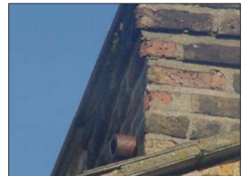
Close up of brickwork, in average condition
