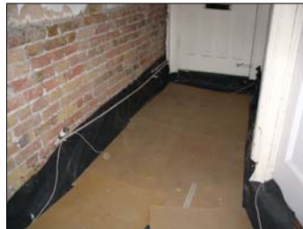
Damp proofing work to the hallway
