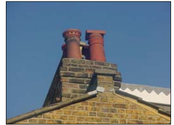
Chimney to both properties
